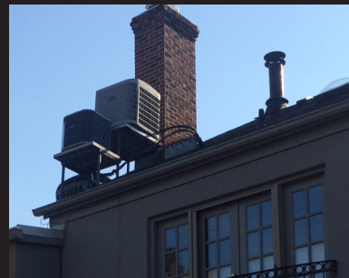
Example of inappropriate unscreened roof-mounted HVAC.
